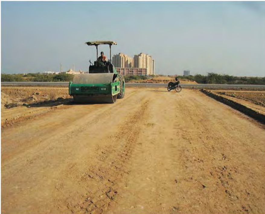
Construction of roads network in Phase-VIII
