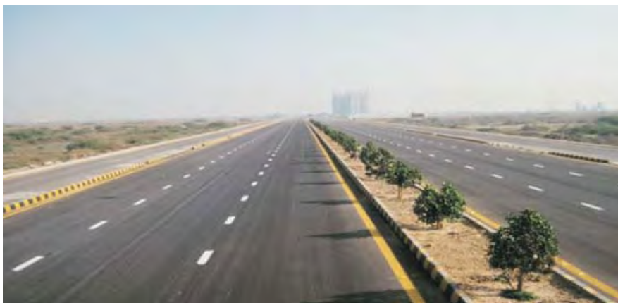
A view of newly constructed roads in DHA Phase-VIII
