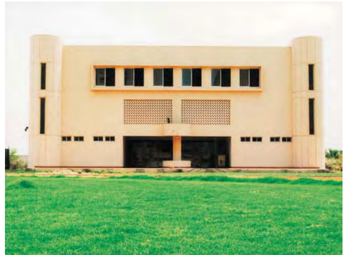
Newly constructed Squash Courts of the Sports Complex
