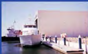
Private Mini Port Complex at Abu Dhabi, UAE
