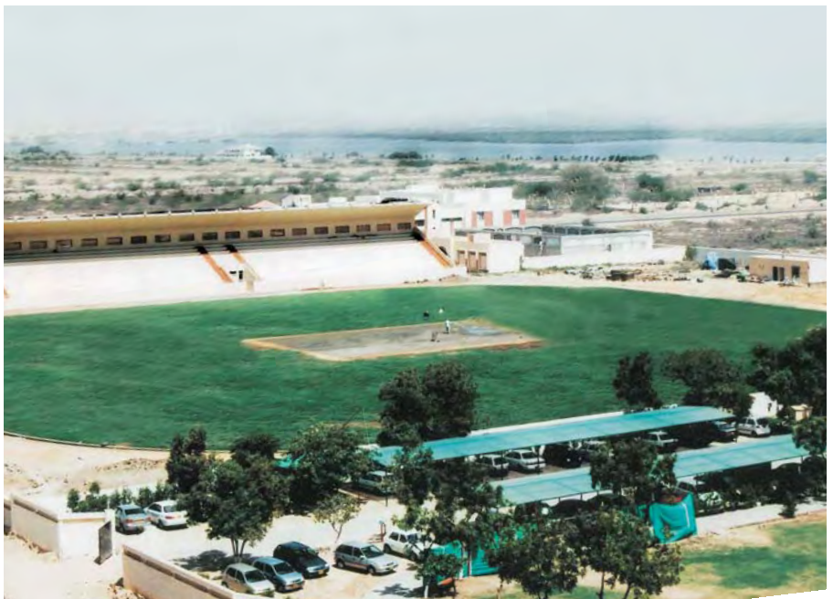
On-going development work at DHA Sports Complex Phase-VIII.
