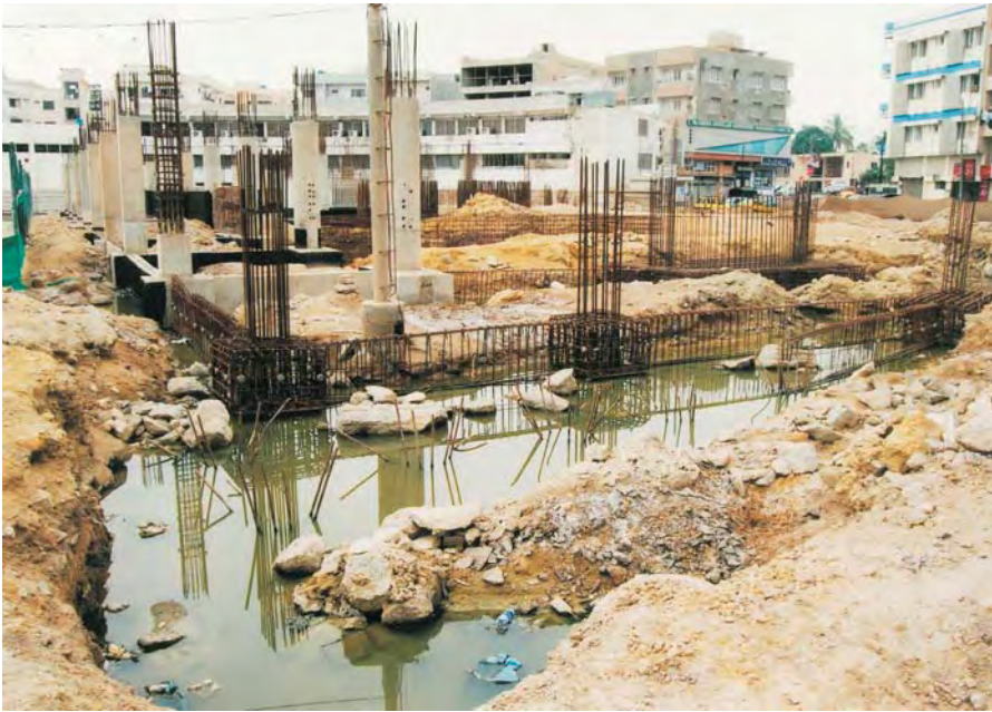
A view of ongoing work of Zamzama Car Parking Plaza.
