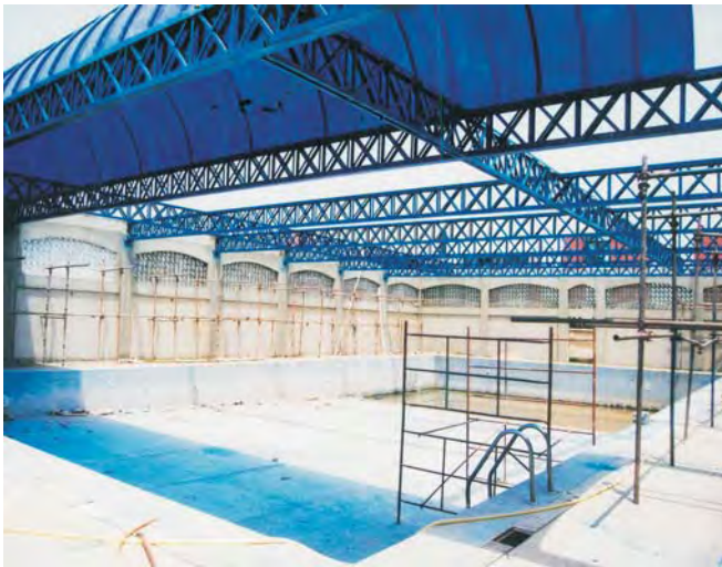
Covered swimming pool at new DHA Sports Complex
