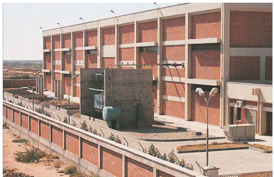
Creek City Grid Station in Phase-VIII.
