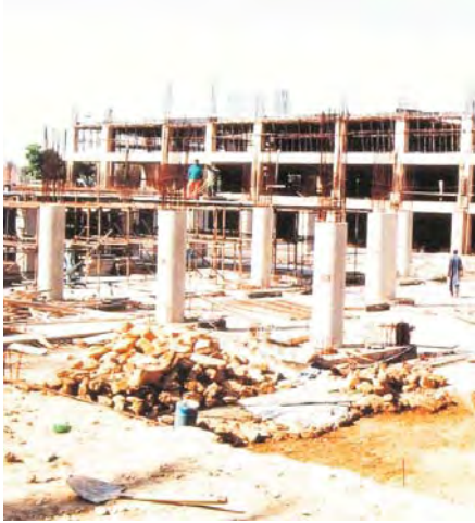
Development of Zamzama Car Parking Plaza in progress
