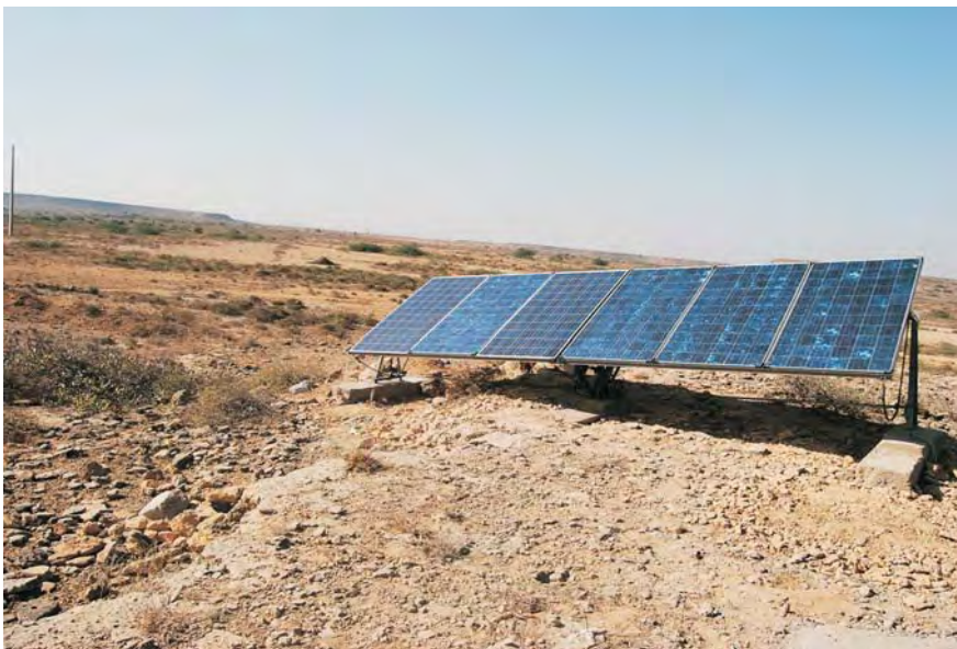
Indigenously built solar panels installed at DHA City site.
