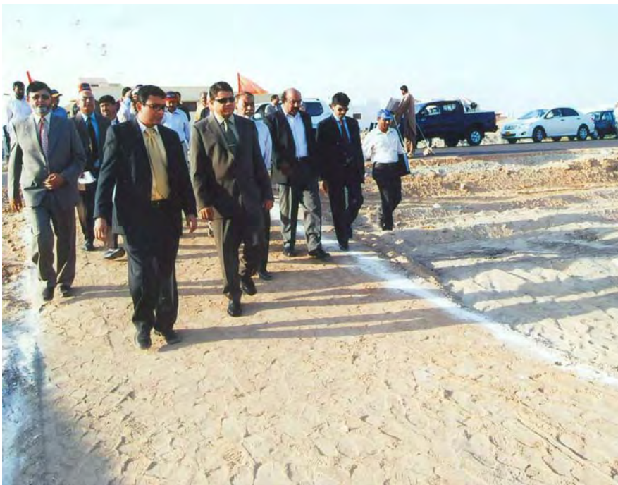
Administrator inspecting the infrastructure development works in DHA Phase-VIII
