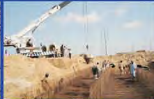
Development works at LDA Hawksbay Scheme-42 Karachi Pakistan
