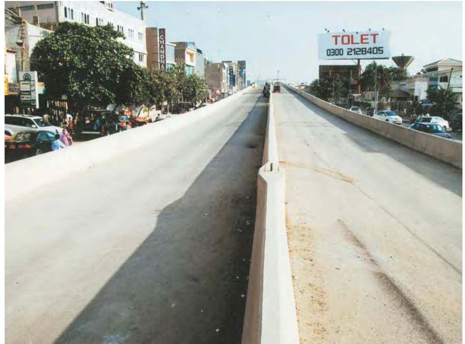
A view of newly constructed Gizri Overpass
