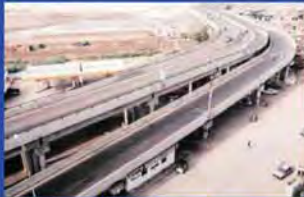
Flyover at Latifabad Railway Crossing, Hyderabad Pakistan
