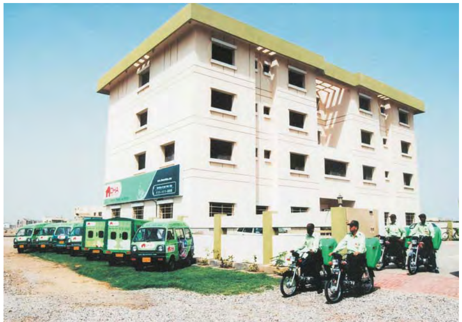
Newly constructed office of DHA Services in Phase-VIII
