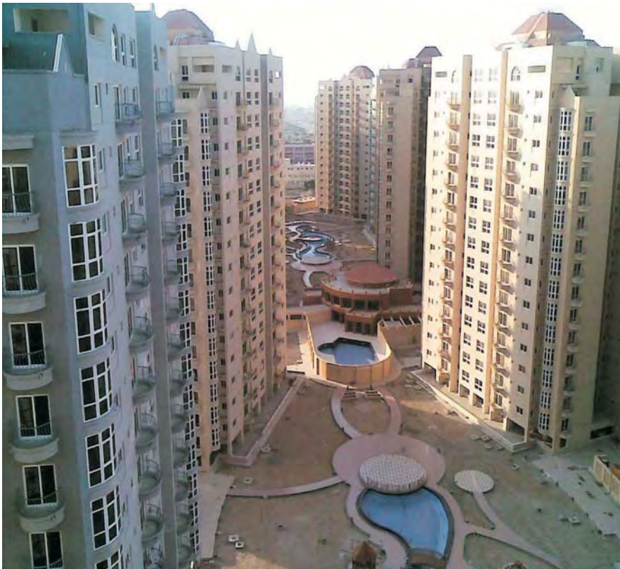
Creek Vistas standing tall under the bright daylight.
