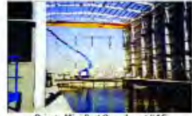
Private Mini Port Complex at UAE
