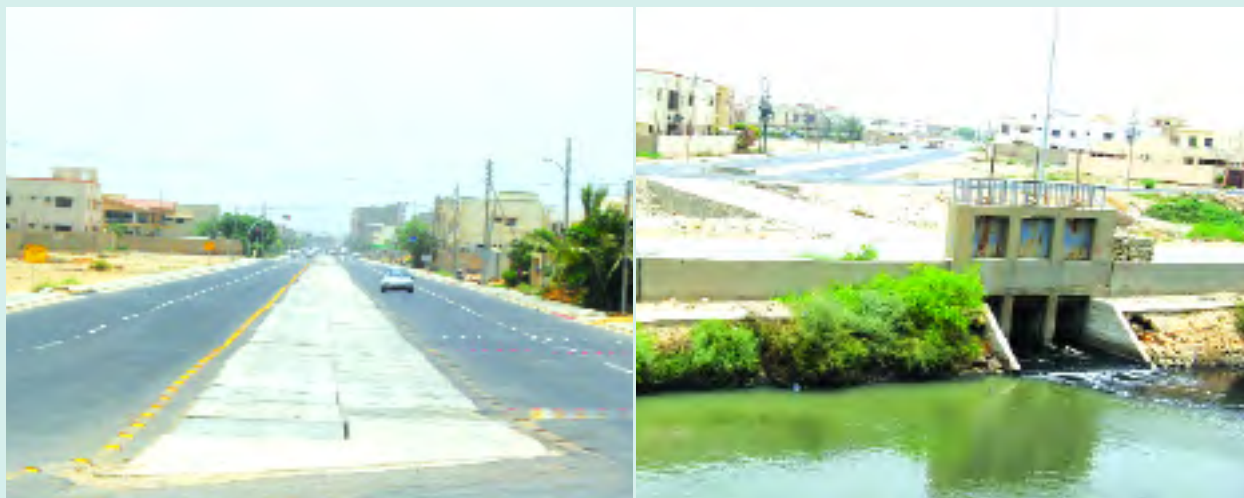
A view showing new Drainage System in DHA
