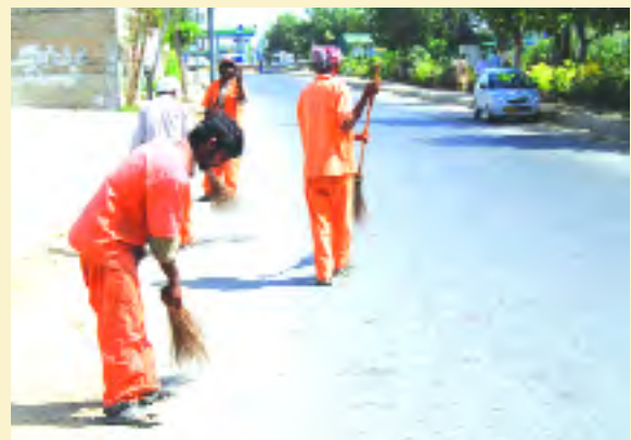
Sweeping of roads in progress
