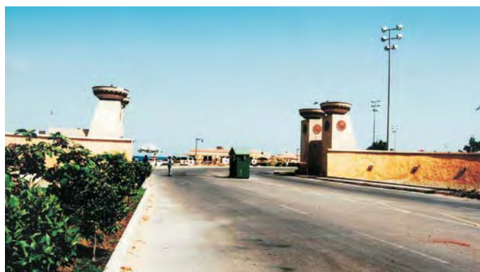
New entrance gate of DA Country & Golf Club
