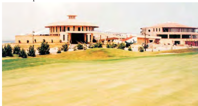
A beautiful view of the renovated Club House.
