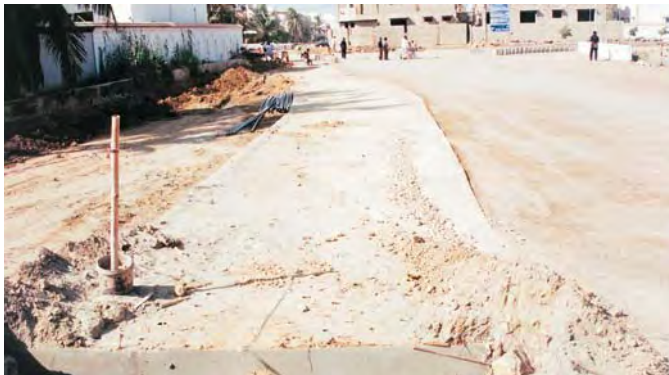
Refurbishment of Commercial Avenue in progress
