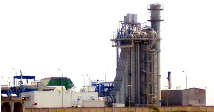
DHA Cogen Power & Desalination Plant.
