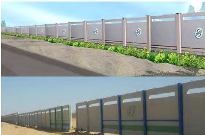
DCK Boundary Wall under construction.
