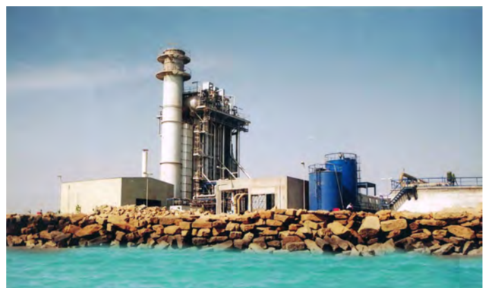
DHA Cogen Plant.
