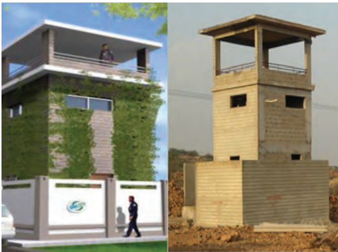
DCK Watch Tower under construction.
