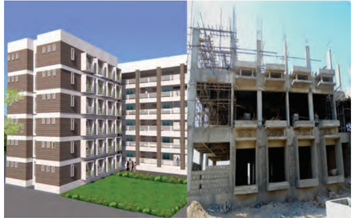
DCK Staff Accommodation under construction.
