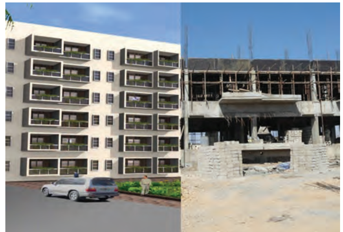
Single Officers' Accommodation under construction.
