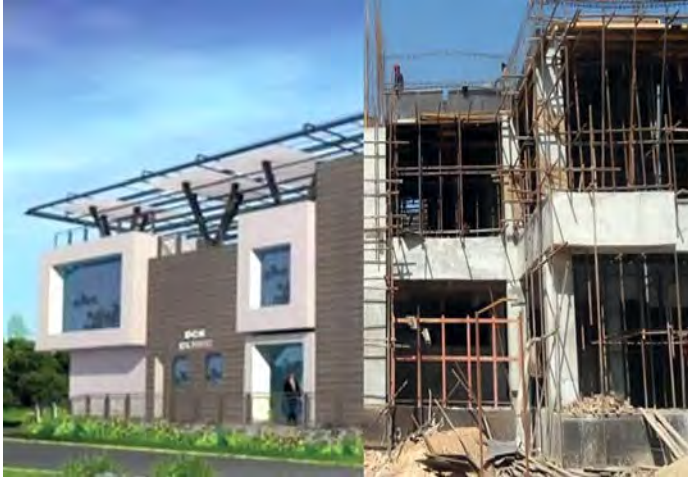
DCK Central Facility Building under construction
