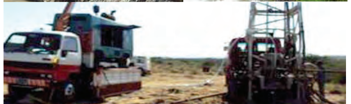
Water Exploration at DCK Site
