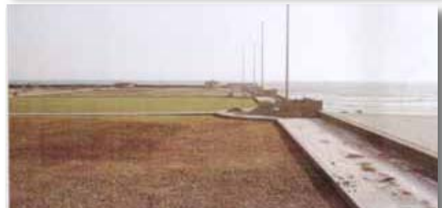
Ongoing Development Works in DHA Phase-VIII
