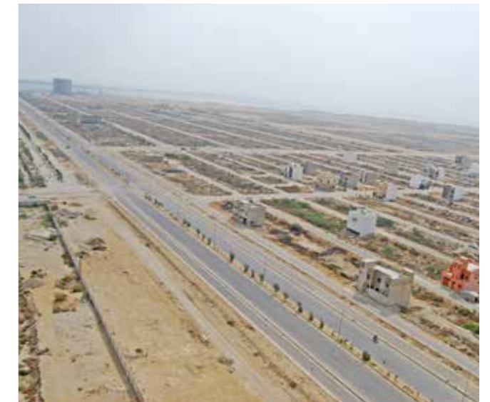
Infrastructure Development Works in DHA Phase-VIII
