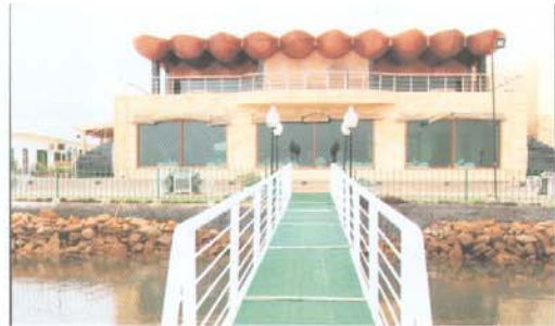
A view of the exquisite exterior of the Club
